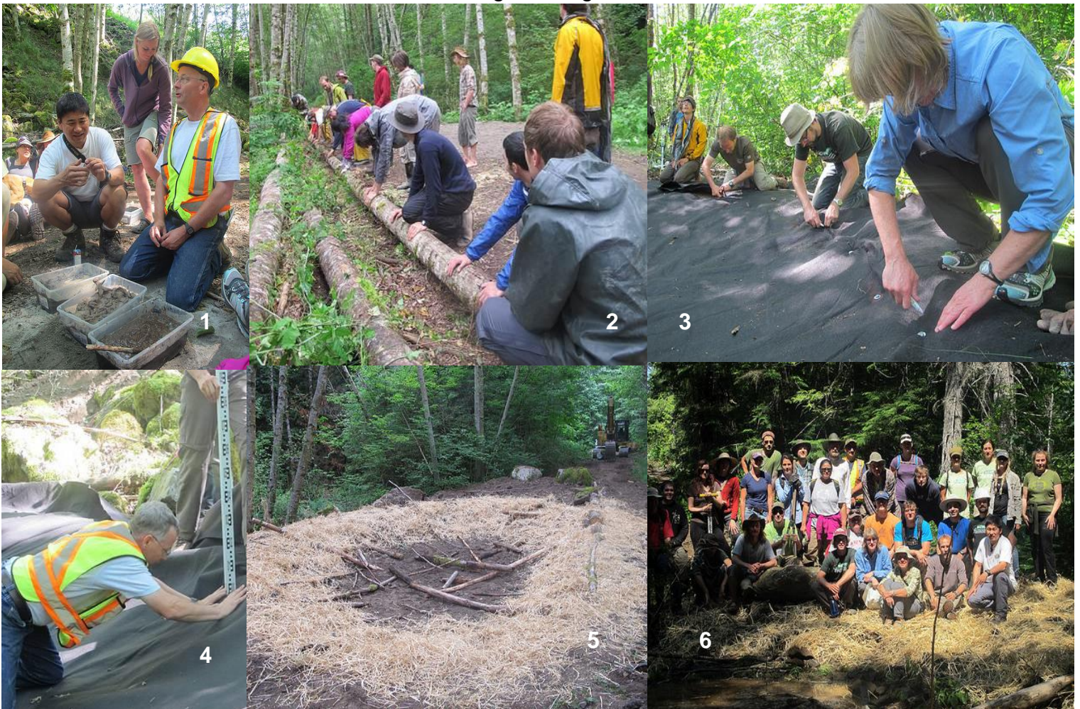
Photo 1. Tom explains the importance of soil types for the construction of wetlands. Photo. 2. Participants creating a path to guide visitors. Photo 3. Trimming the excess liner. Photo 4. Marking the exact place for pegs. Photo 5. Where there was road, there are wetlands. Photo 6. The group after completing construction.
