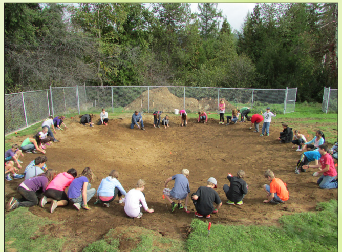
A class is taken outside for some hands-on wetland construction at the Kinnaird Elementary School in Castlegar. Here the BCWF guides the group in removing rocks before the liner is installed.
