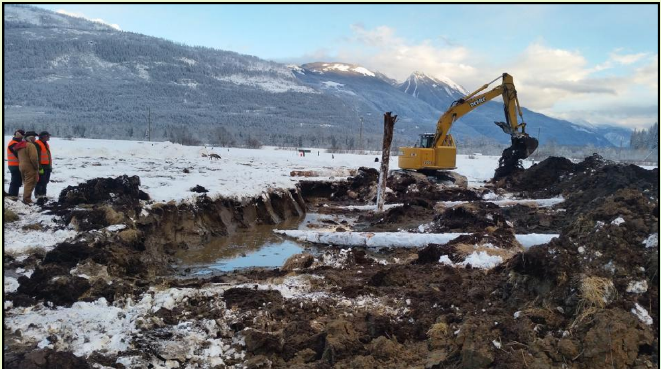
Constructing wetlands in January allowed the excavator move across what is otherwise saturated fields.
