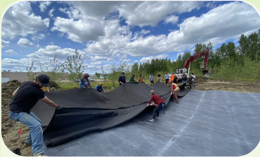
Students laying out the wetland liner at Mackenzie Secondary School.
